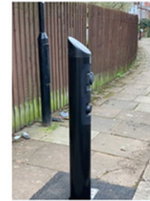
Image of charging bollard
